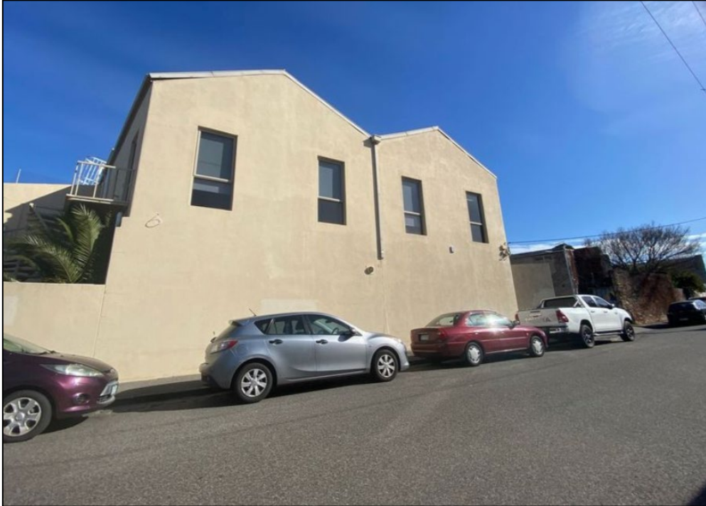
Figure 8 The central courtyard connected to a vehicle crossover accessed from Canterbury Place (view from Canterbury Place)
