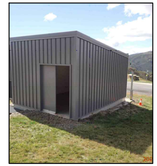
PHOTO TAKEN FROM SOUTH OF SITE
