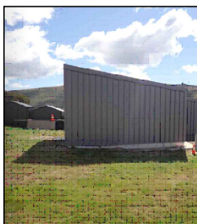
PHOTO TAKEN FROM SOUTH-EAST OF SITE
