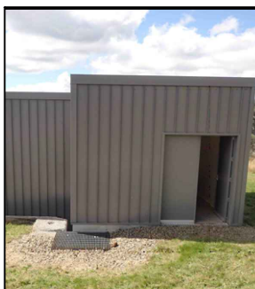
PHOTO TAKEN FROM SOUTH-WEST OF SITE
