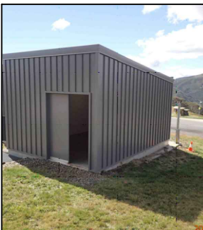
PHOTO TAKEN FROM SOUTH OF SITE
