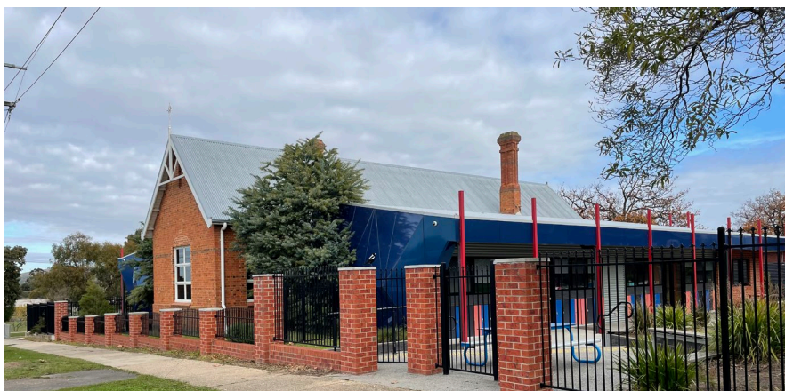
Figure 3 , Existing condition of former St Mary's School building (May 2023)
