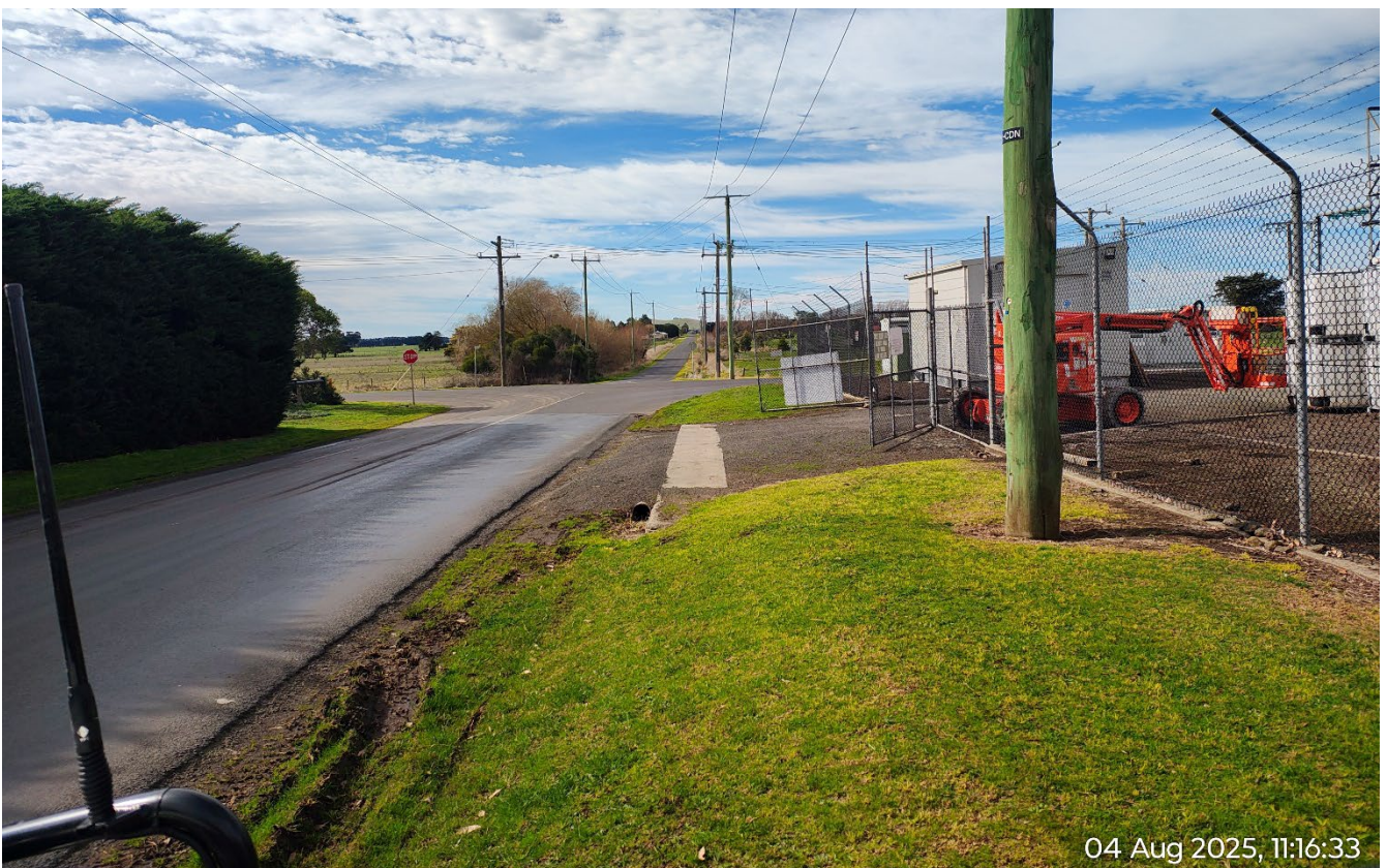
Image 2D. East up Wiridgil Road from the Sub-station on Camperdown-Lismore Road (Abzeco 04/08/2025)
