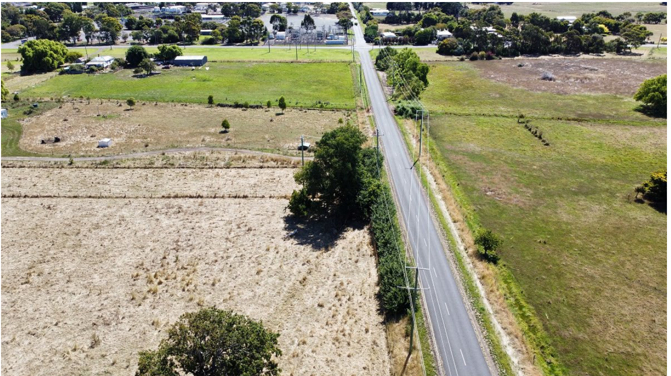
Image 2C. Roadside vegetation on Wiridgil Road down to the power sub-station on Camperdown-Lismore Road (Abzeco 10/02/2023)
