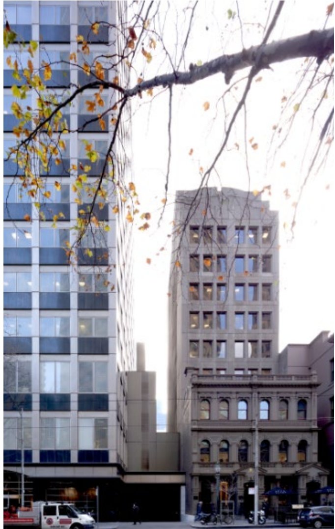
Picture 2 No. 60 & No. 52 Collins Street, Melbourne
