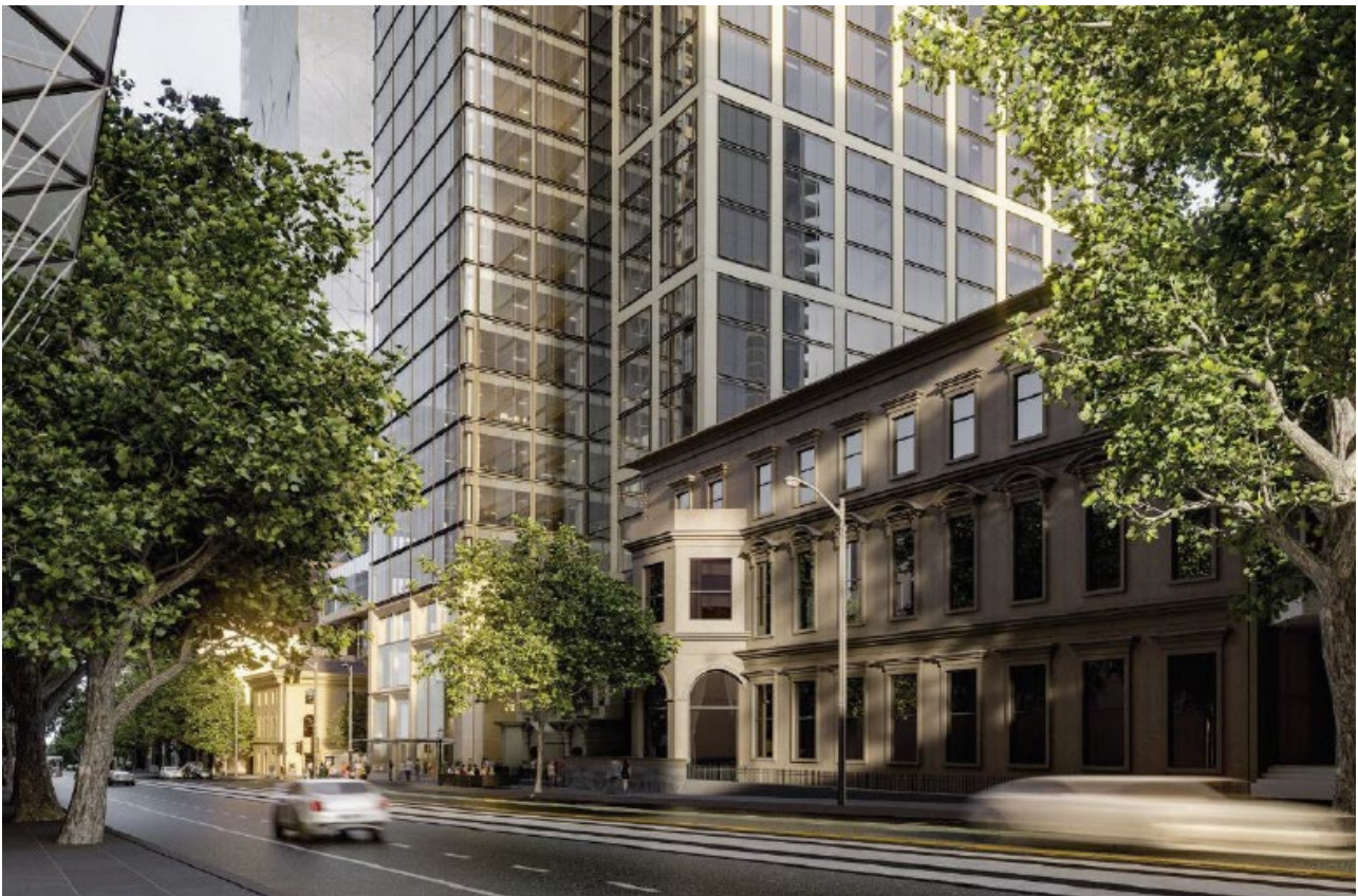
Figure 6 Proposed Development viewed on Collins Street, with the existing Melbourne Club to the East
