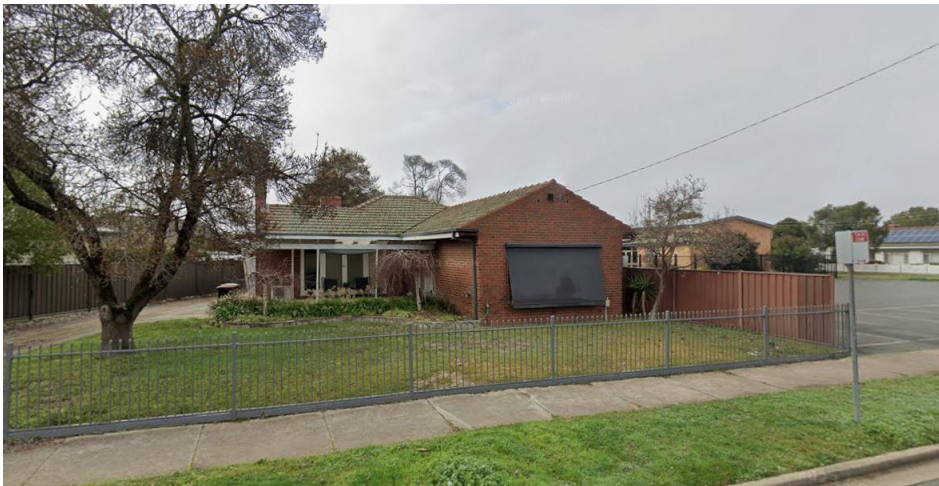
Figure 3. 11 King Street (source: Google)
