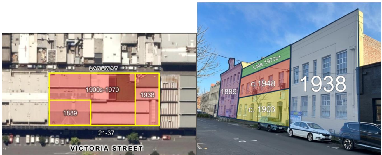
Figure 27 Annotated aerial and streetscape view showing periods of construction (Heritage Impact Statement)
