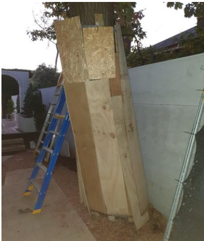
Example: Trunk protection. Timber boxing around the tree trunk
