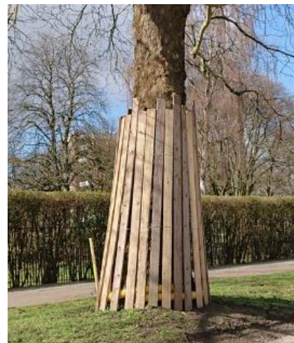
Example: Trunk protection. Timber battens around the tree trunk
