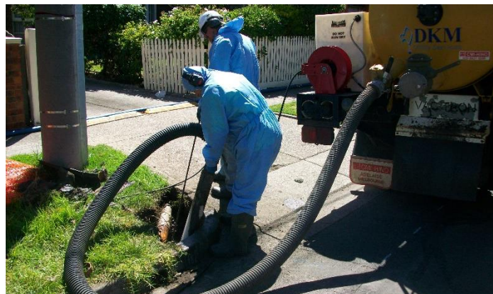
Photo: Non-destructive digging (NDD) using a Hydro Vac / excavation vac
