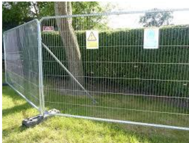
Example: Temporary fencing. Tree Protection Fencing
