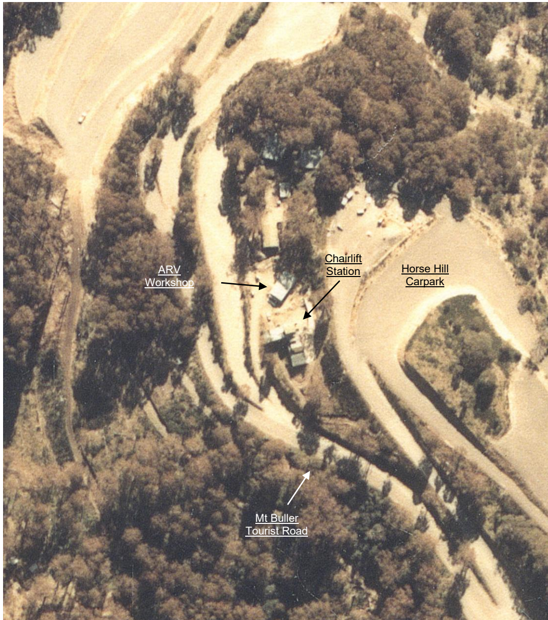
Horse Hill Carpark and Northside Express Chairlift Bottom Station Area – April 1985
