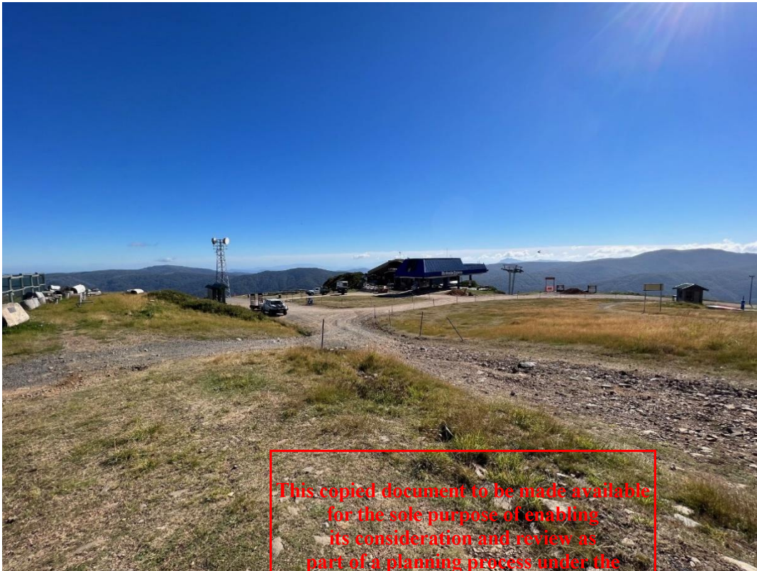
Image 1: Looking north to the top station works area
