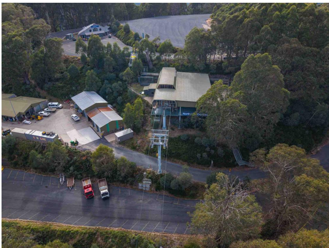
Image 3: Looking east to the bottom station works area
