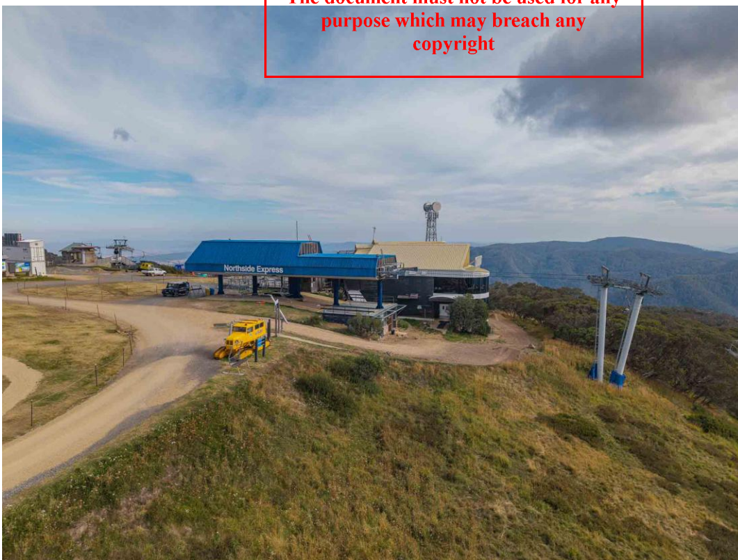
Image 2: Looking northwest to the top station works area
