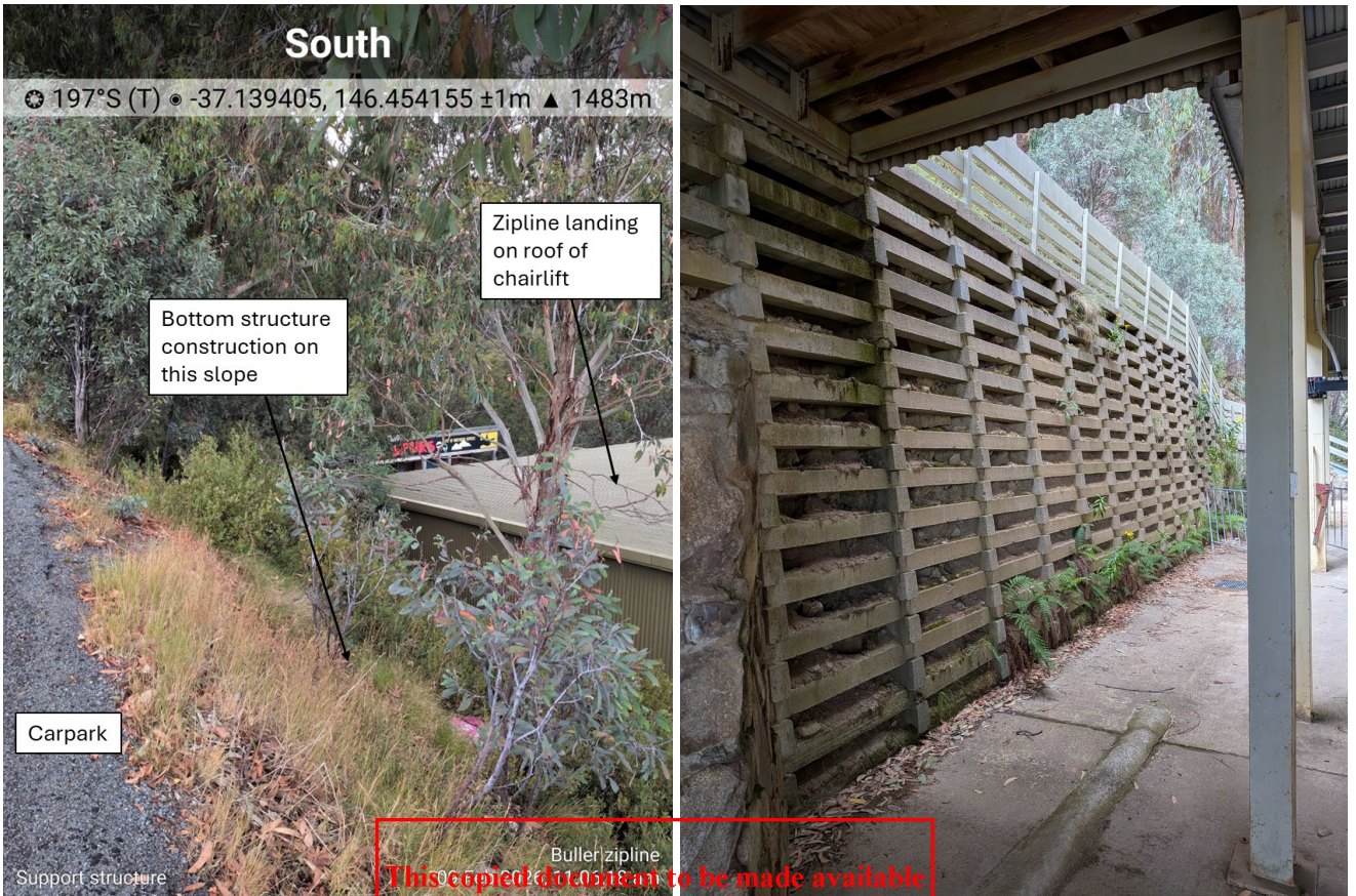
Figure 4 Left – location of zipline bottom structure. Right – crib wall at base of slope.
