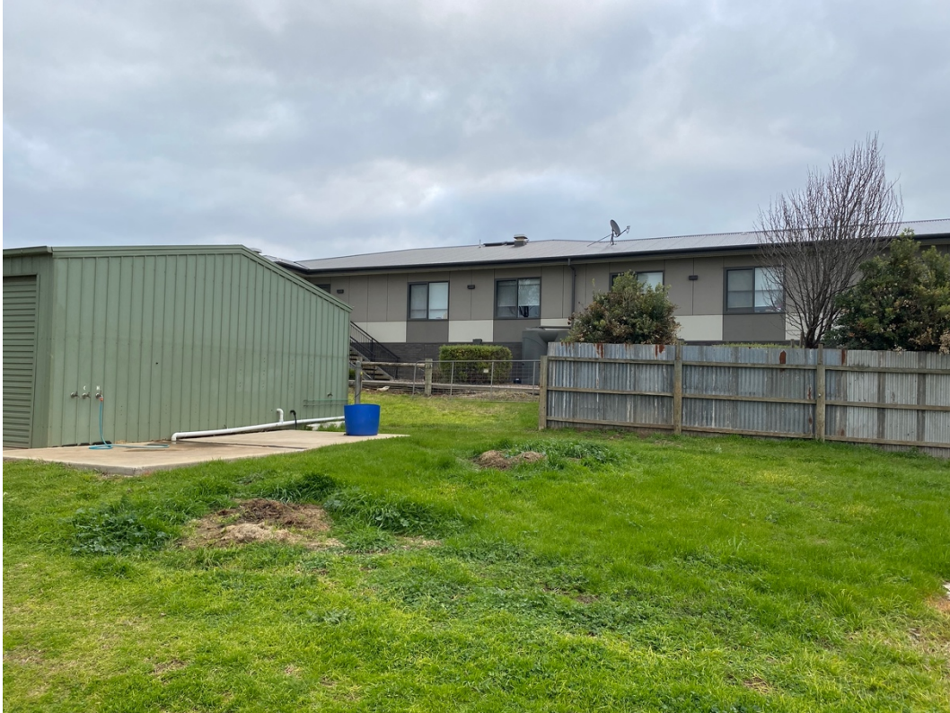
Image 9: Westerly view towards adjoining residential units
