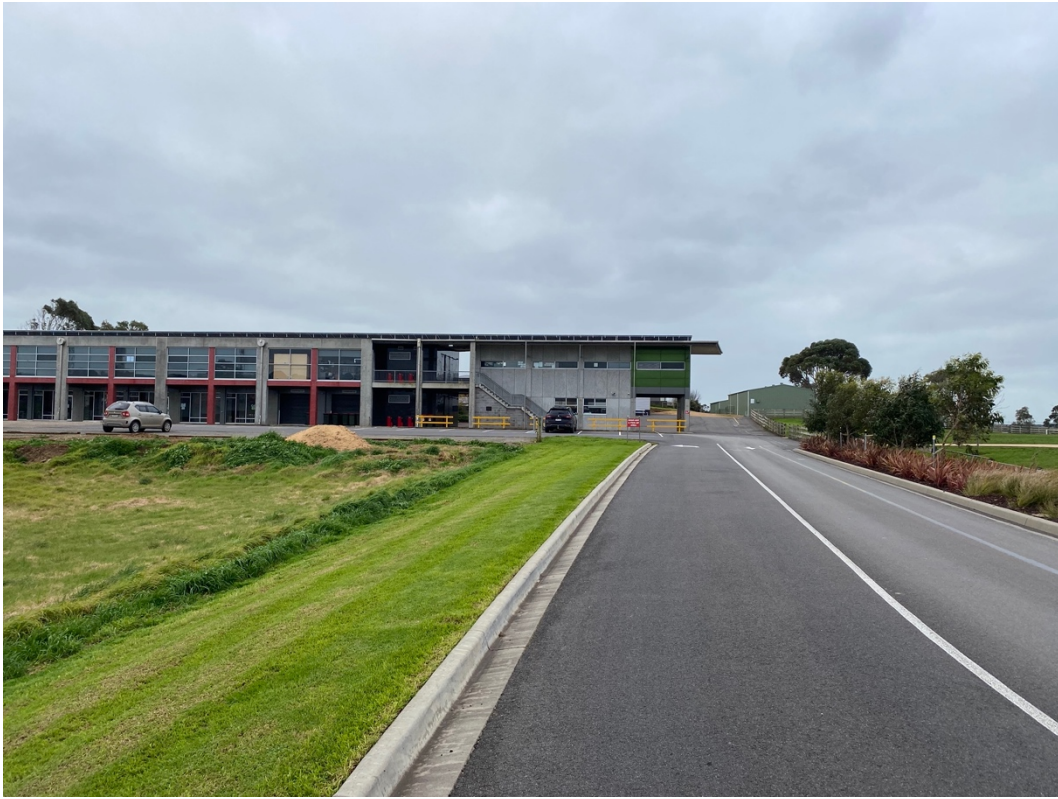
Image 3: View looking north towards existing 'G Block'
