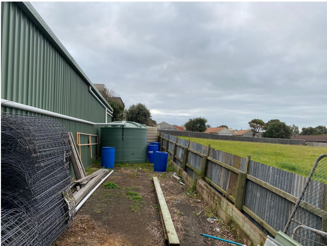
Image 10: Existing sheds and fence to be demolished in Year 9 Centre proposed location
