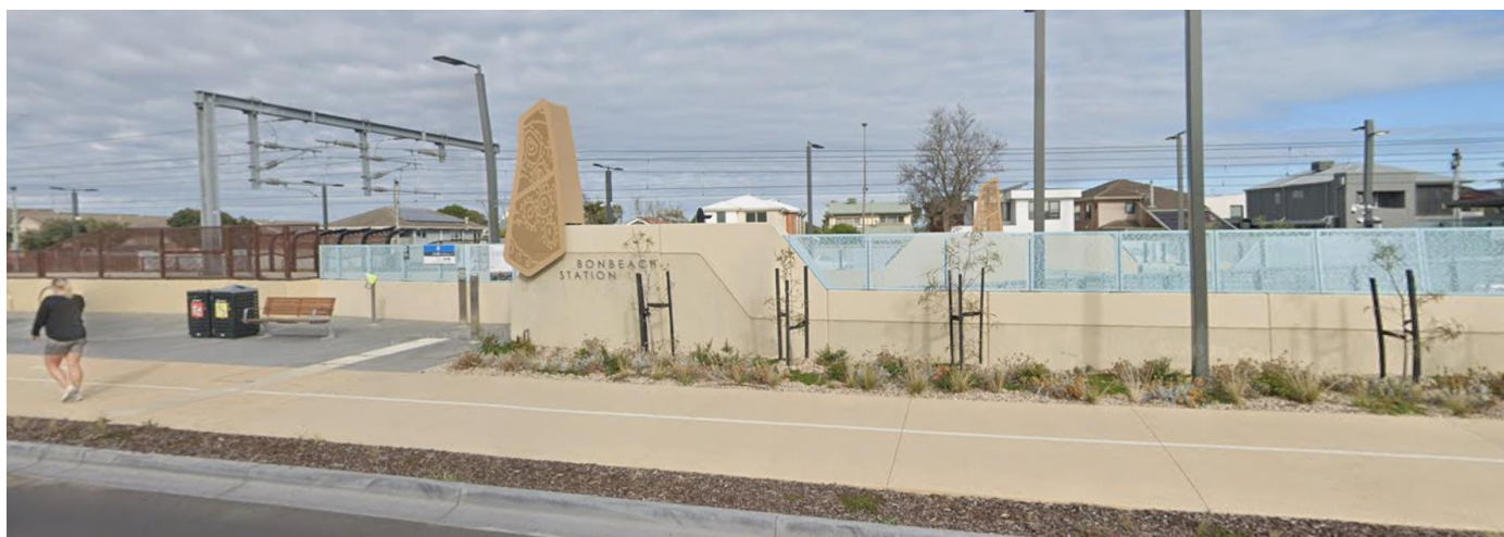
Above: Street view of Bonbeach Station, to the west of Station Street.
