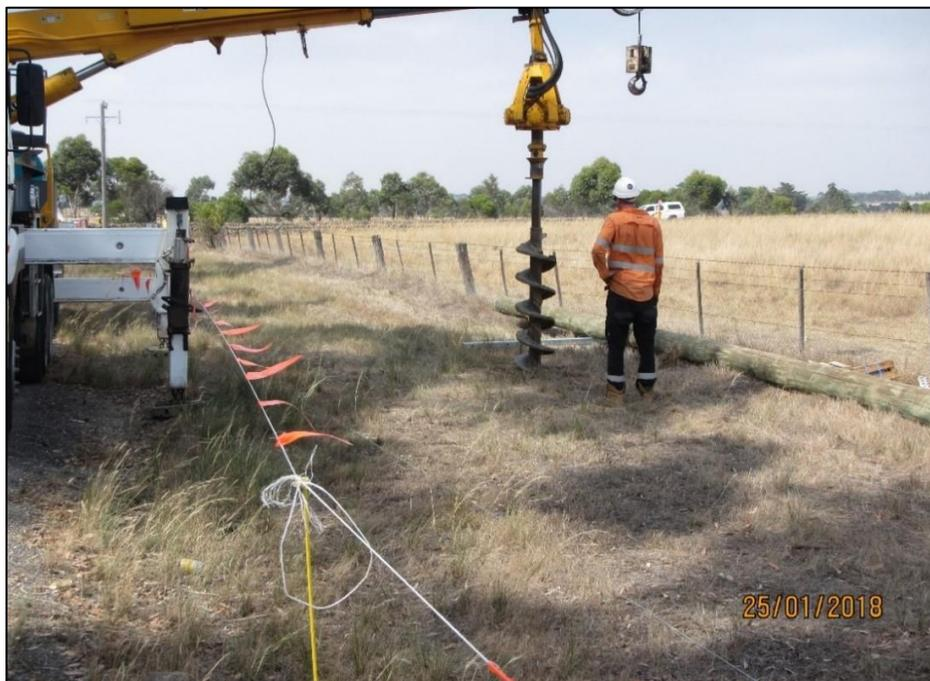
**Figure 4: Example of hole being augured via arm from truck (note in this example the roadside vegetation was deemed to be native in places and fencing was set up to keep the truck from the shoulder)**
