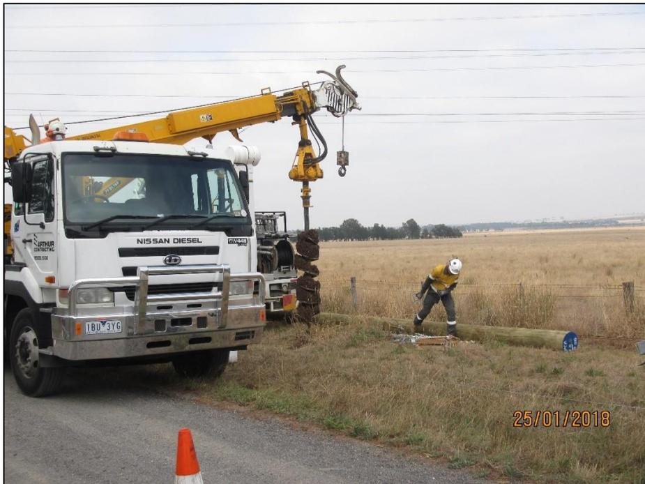
**Figure 3: Example of a hole being augured via arm from truck (note in this example the roadside vegetation was deemed to be non-native, hence the truck parking slightly on the verge and the other truck in the background)**
