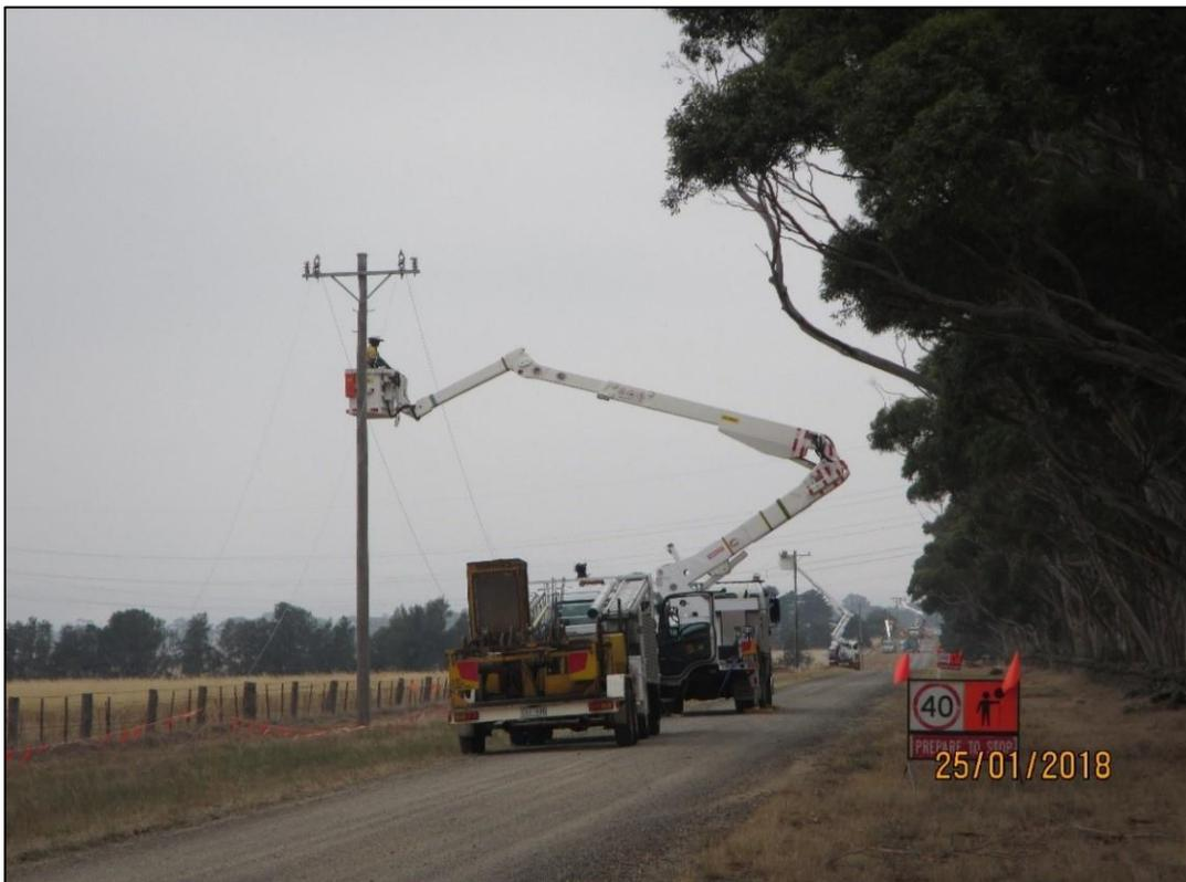
Figure 6: Example of contractors working on the new or replacement installation. Note the truck is still in the road carriageway
