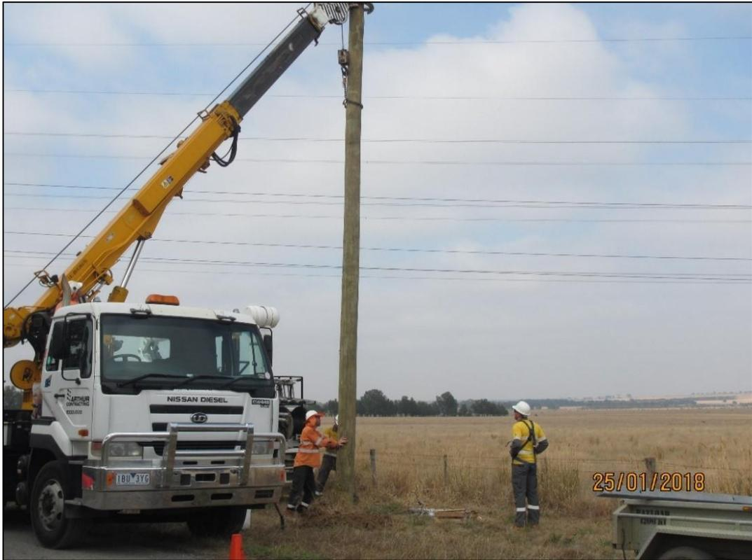
Figure 5: Example of pole being installed via truck crane
