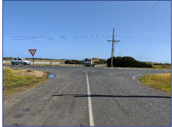
Figure 7: Churchill Road (view south)
