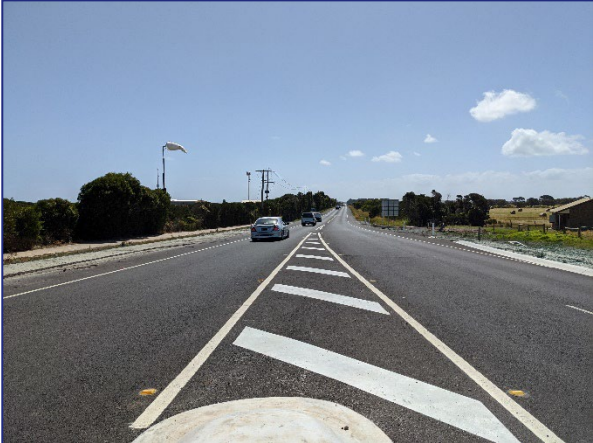
Figure 5: Phillip Island Road (view west)
