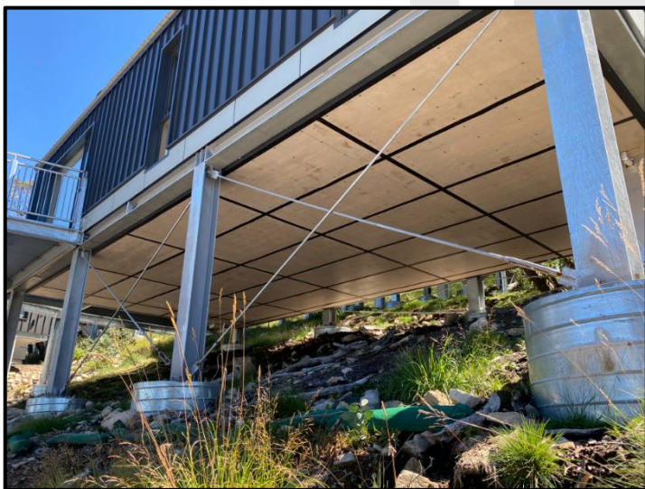
Photo 6 View of sub-floor area beneath the subject building.
