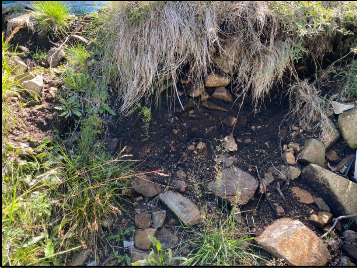
Photo 4 view of typical insitu soil/rock profile exposed in a site cut at the south-eastern corner of the subject site.
