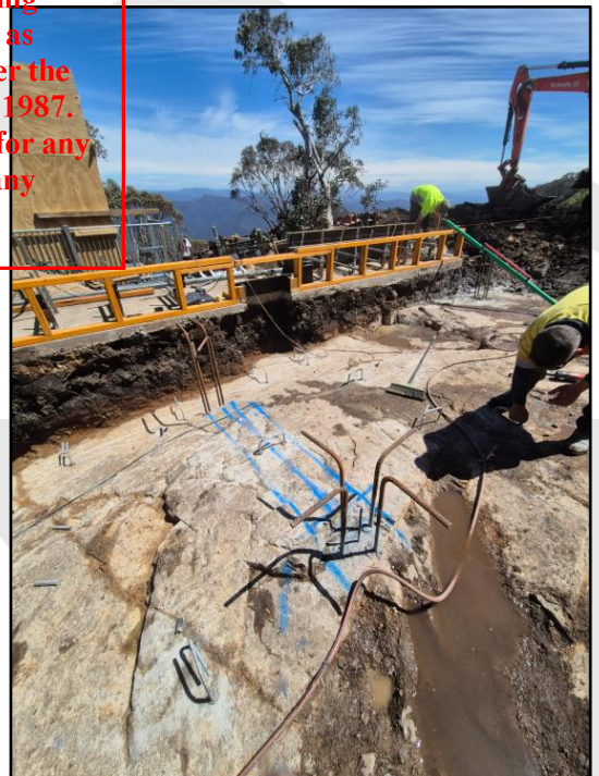
Photo 3 (previously taken by contractor) of insitu, slightly weathered granodiorite bedrock exposed in the footing excavations for a nearby building.
