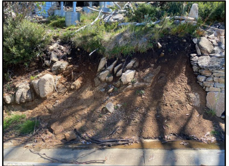
Photo 5 view of typical insitu soil/rock profile exposed in a site cut above Whitehorse Village Road near the south-western corner of the subject site.
