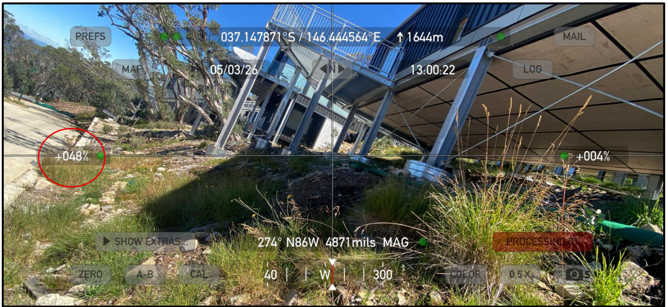
Photo 1 view of typical degree of slope on road CUT embankment (taken on angle to match the slope).
