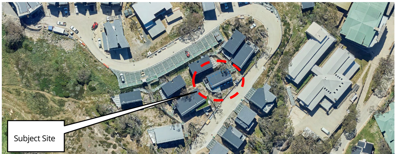
Figure 7: Ariel image of site
