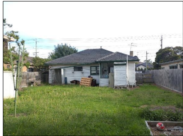
822 Centre Road rear yard as viewed from south
