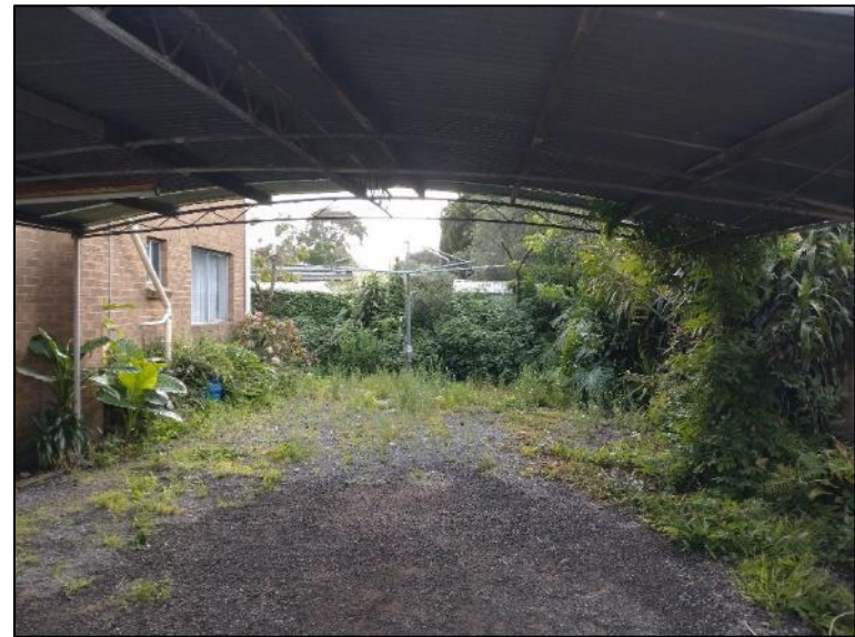
820 Centre Road carport and rear yard as viewed from west
