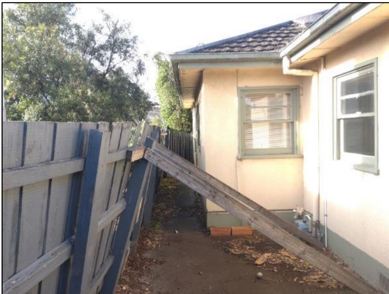
824 Centre Road eastern boundary as viewed from north
