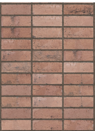
BR2 Existing Heritage Brick as Paving
