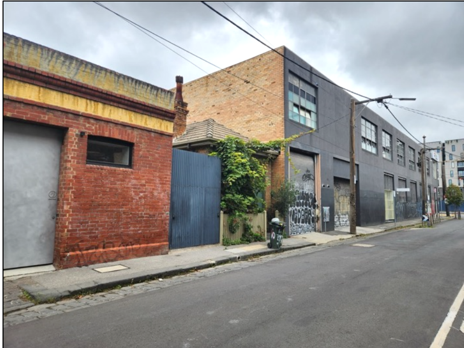
Figure 15 View west along Argyle Street, with 12 Argyle Street at left, single storey Victorian house at 10 Argyle Street, centre, and heavily altered interwar factory at right.
