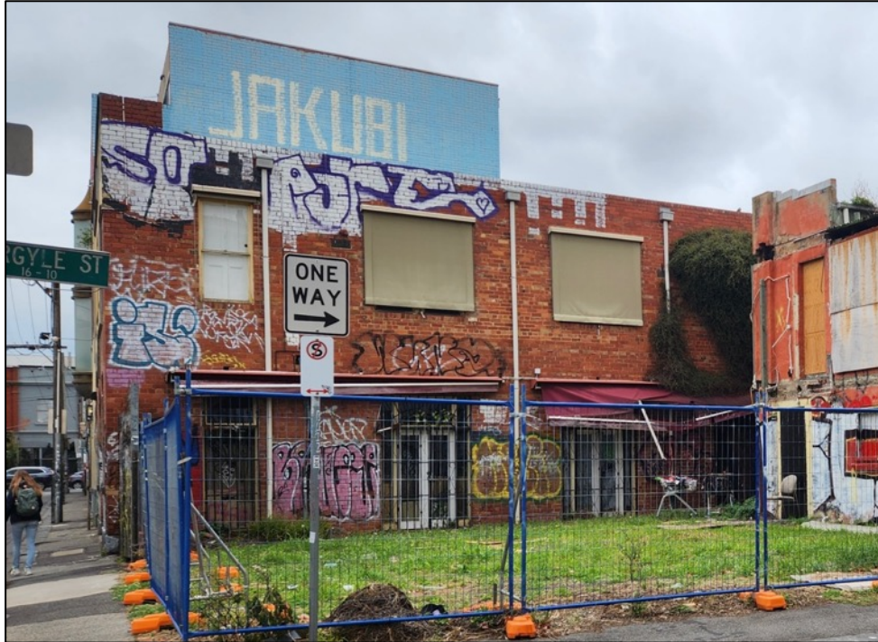
Figure 8 The northern (side) elevation to the former stable has received modern openings at ground and first floor.
