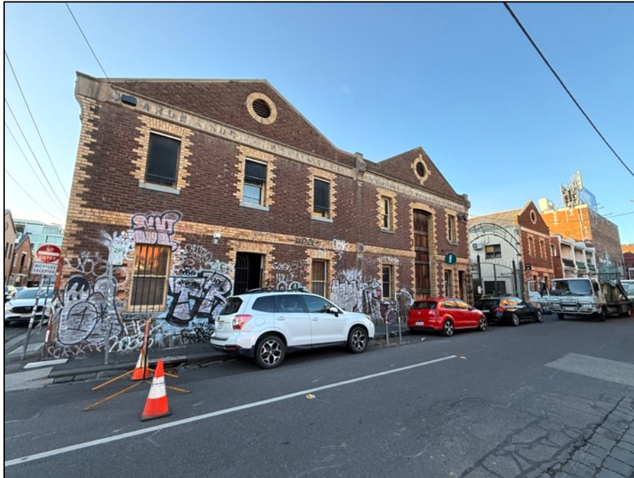
Figure 14 The Former Harrison's Cordial Factory (VHR H2257) at 14-16 Spring Street, opposite the subject site to the east.
