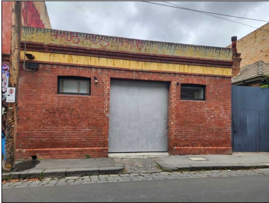
Figure 12 Frontage of 12 Argyle Street, former stables building, that was part of the Spring Street stables site in earlier years.
