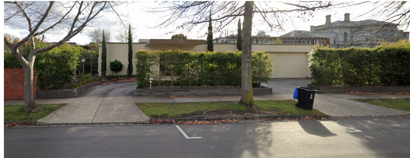
1. View from Heyington Place
