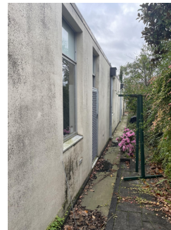
4. View of south boundary
