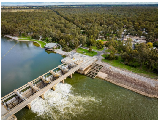
Figure 1912: Torrumbarry Wier and Holiday Park
