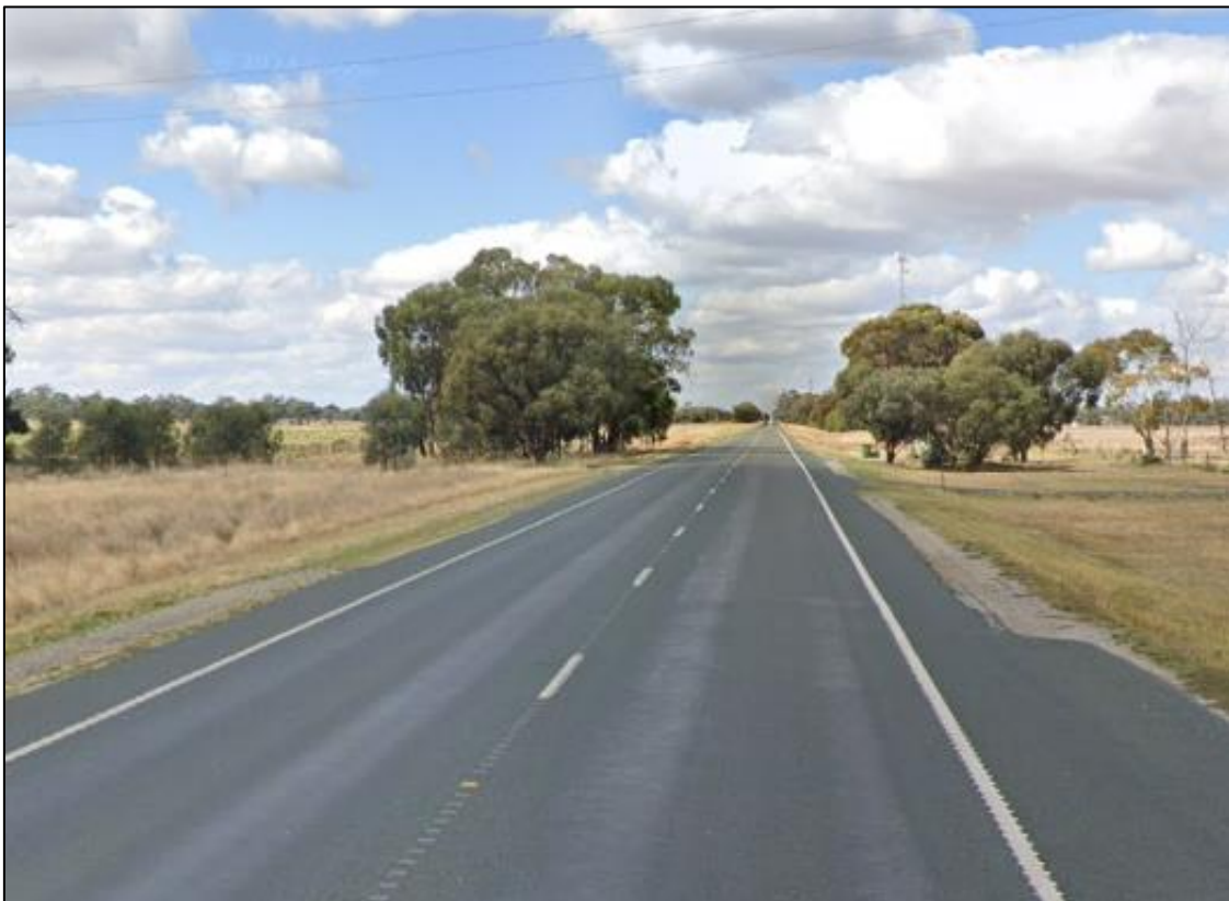
Figure 4-2: Murray Valley Highway (facing east from Davis Road)
