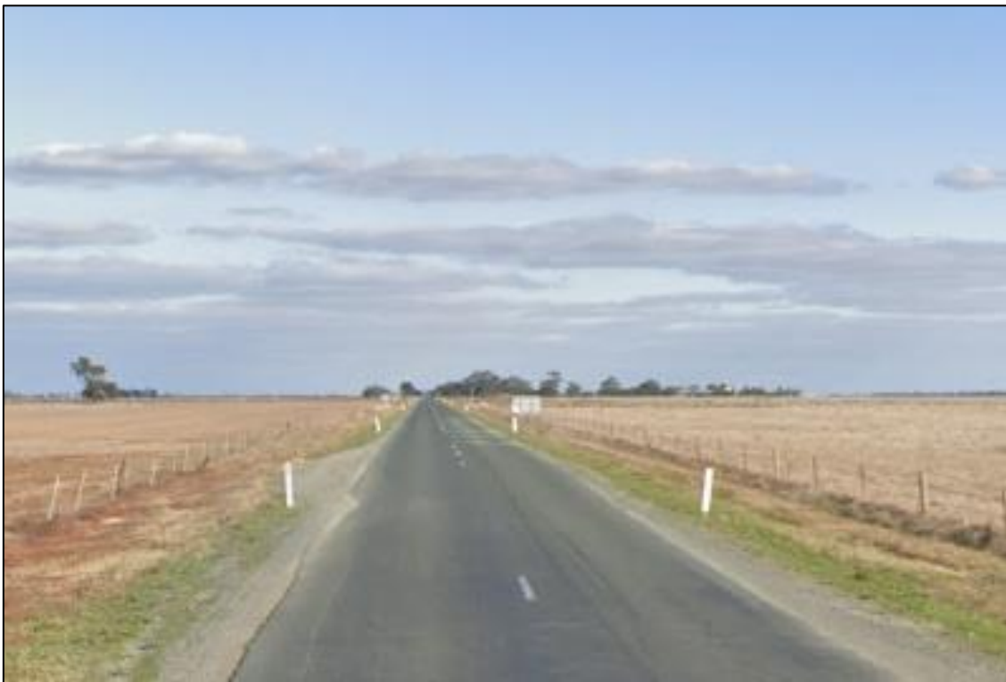
Figure 4-3: Roslynmead Road (looking south from the Murray Valley Highway)
