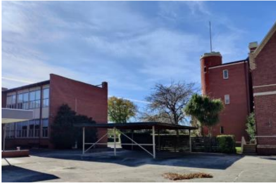
Figure 18: View of the northeastern corner of the site. The modern Year 8 Building and freestanding shelter are in the left, and the Convent building in the right. Source: Trethowan Architecture, 2023.
