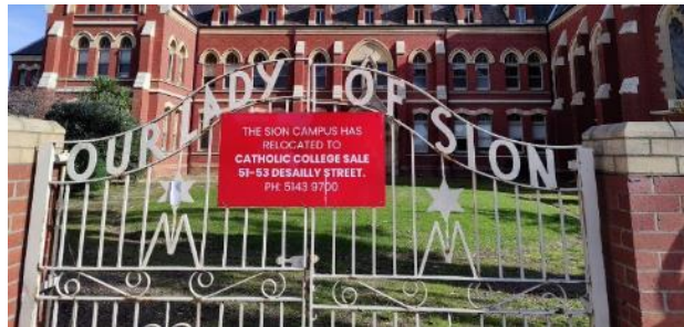
Figure 3: View of the east entrance gates and the Convent building in the background. Source: Trethowan Architecture, 2023.
