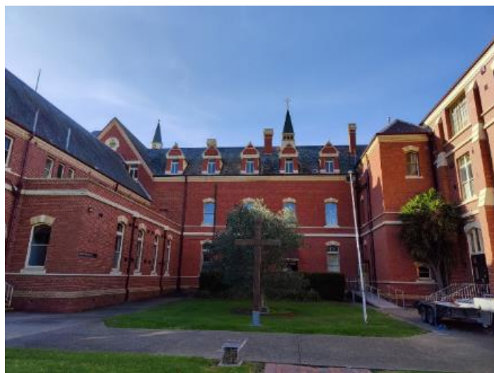
Figure 17: View of the Convent building's west courtyard. A large timber cross is observed in the centre. Source: Trethowan Architecture, 2023.
