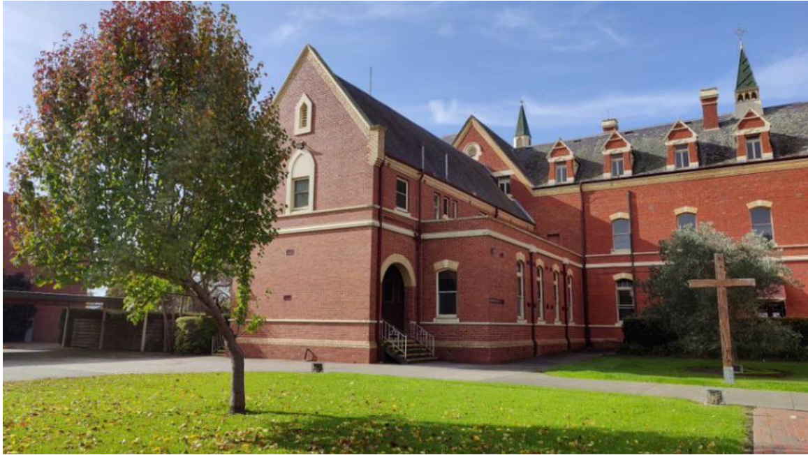
Figure 10: View of the 1953 portion of the North Wing from the west lawn. Note the flat-roofed structure with an accessible outdoor area abutting its south. Source: Trethowan Architecture, 2023.
