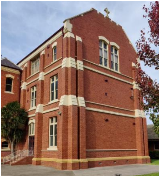
Figure 11: View of the north and west façades of the South Wing. Source: Trethowan Architecture, 2023.
