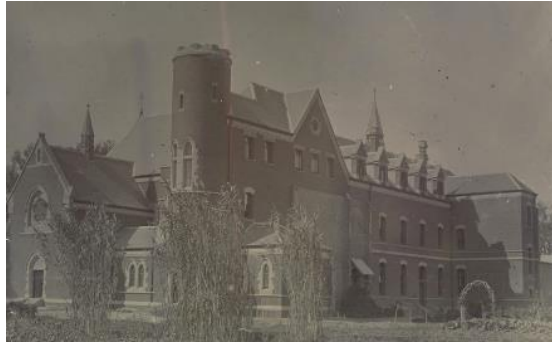
Figure 27: View of the north and west façades of the Convent building. Note the absence of the north and South Wings, indicating the photo was taken prior to 1938. A section of wall appears to have been infilled. Source: State Library of Victoria.
