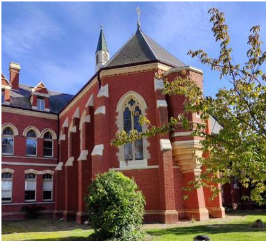
Figure 8: View of the east façade of the 1901 North Wing chapel. Source: Trethowan Architecture, 2023.
