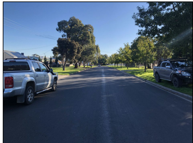
Figure 6 Codrington Street facing west
