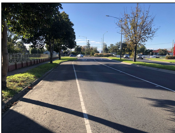
Figure 9 York Street facing north
