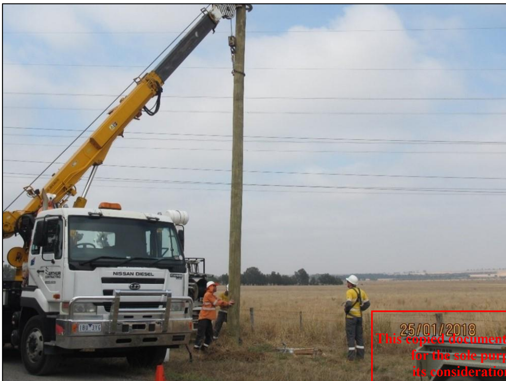
Figure 9. Example of pole being installed via truck crane
