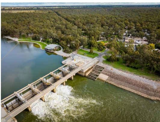
Figure 1912: Torrumbarry Wier and Holiday Park
