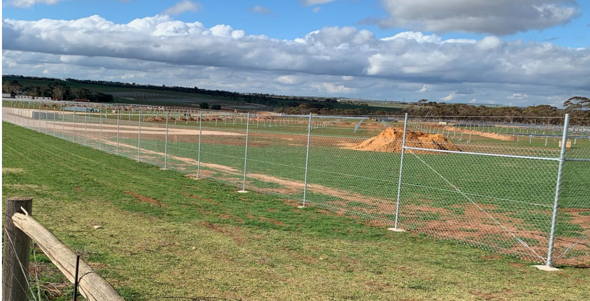
Fig 25. Typical solar farm perimeter fence (Approx. 2.3m high) source: Tetris Energy, Mannum Solar Farm
