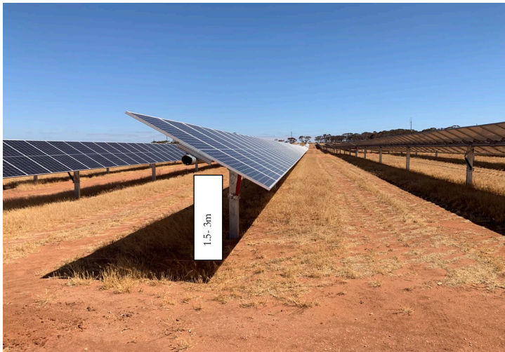
Fig 14. Example of a Single Axis Solar PV Array (Source: Tetris, Mannum solar farm)
