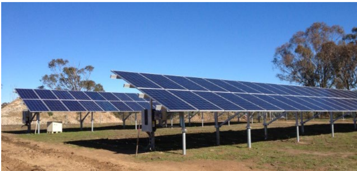
Fig 1. Example Solar PV Array – screw mounted
