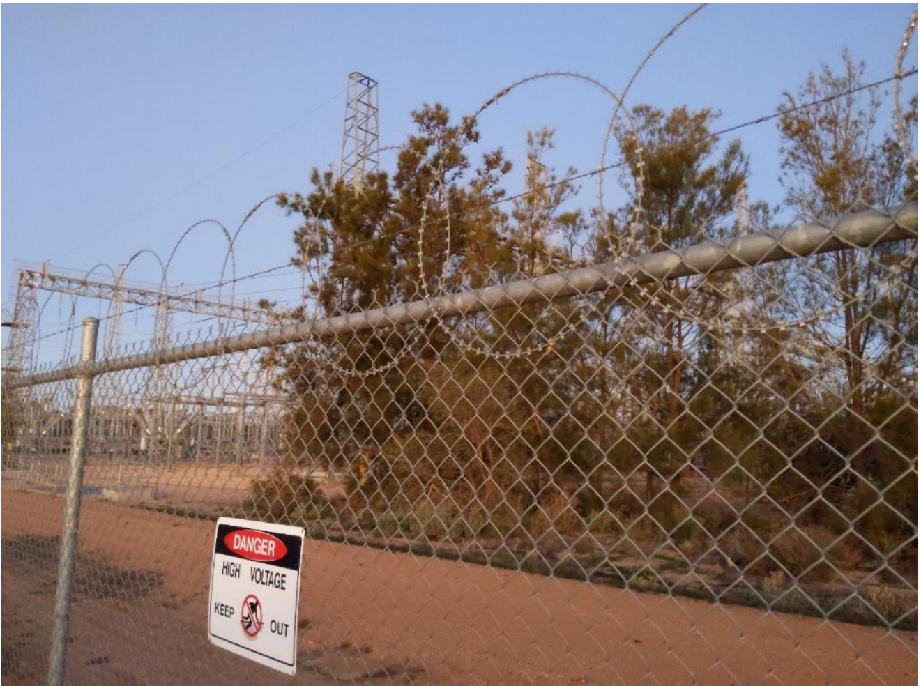
Figure 3.11 Semi-arid Chenopod Woodland within the substation (July 2020)
