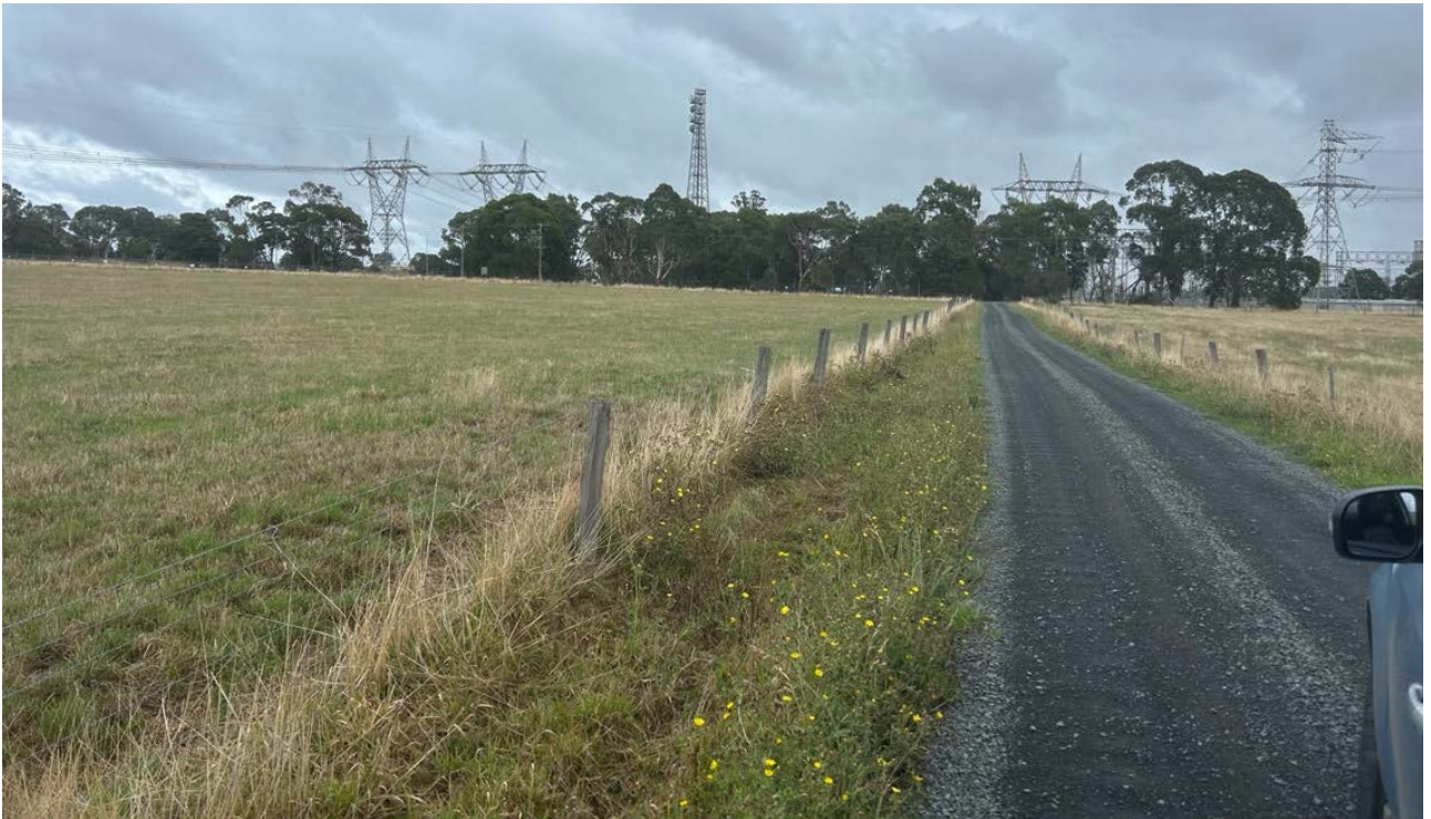
Figure 4-3: View from driveway towards Tramway Road and the Hazelwood Terminal Station
