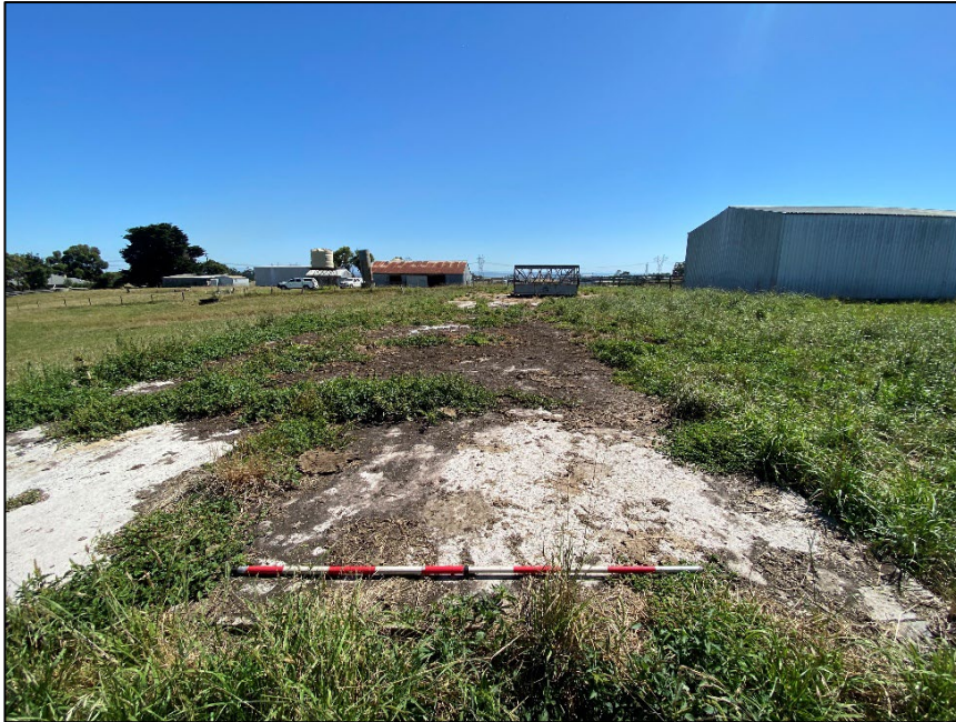
Plate 3: Concrete conglomerate foundations, looking north
