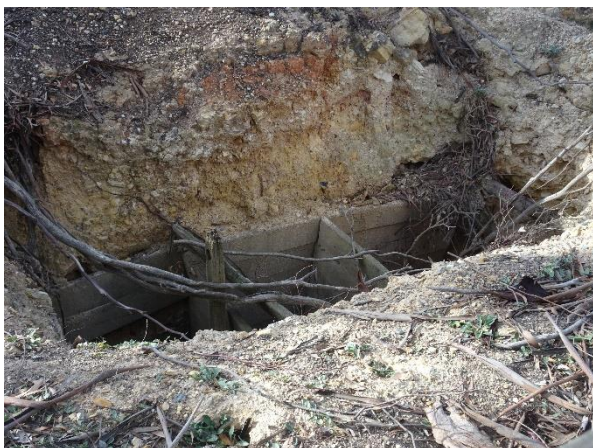
The three compartment shaft retaining extensive timbering
