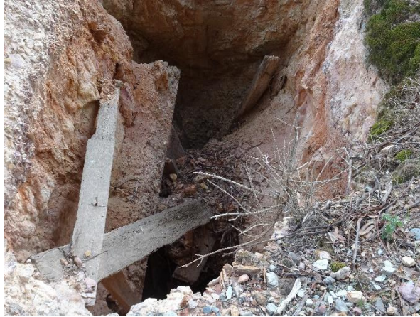
Detail of shaft and timbering
