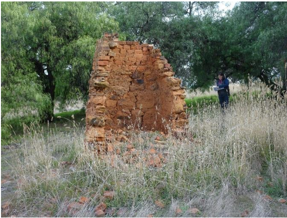
Remnants of stone and timber (?) cottage, with random rubble stone chimney, some loose bricks. Enclosed in a 'grove' of peppercorn trees, some in a line suggesting a windbreak planting.
