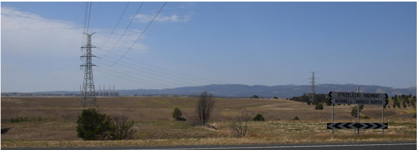
Figure 6-10: Landscape Unit 3 – Industrial/Mining example (Transmission Line)
