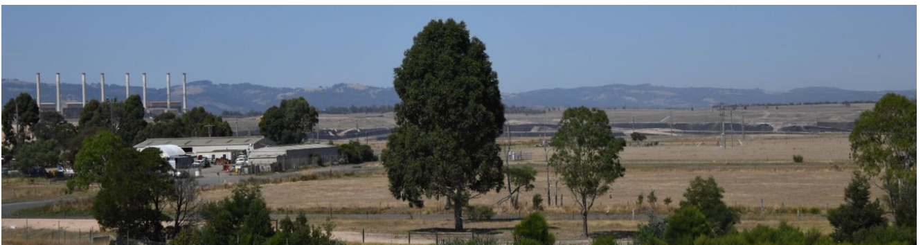
Figure 6-9: Landscape Unit 3 – Industrial/Mining example (Hazelwood Power Station)
