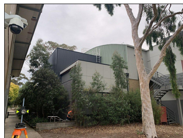
PHOTO 8 - NORTHWEST CORNER OF SUBJECT SITE FACING SOUTHWEST FROM CONCRETE PATH
