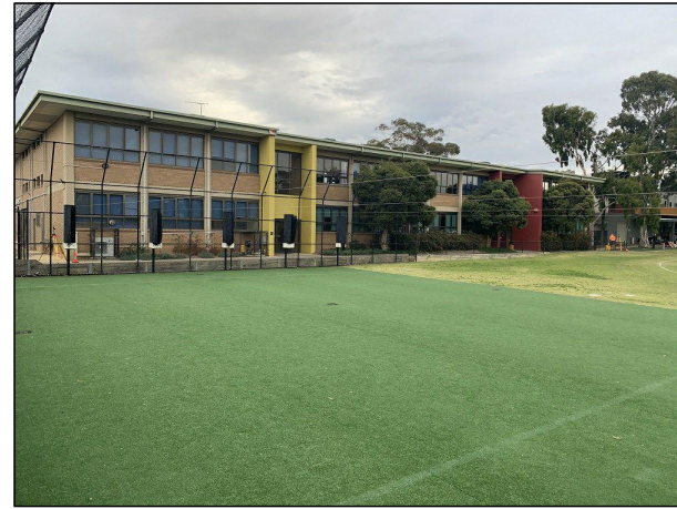
PHOTO 1 - NORTHEAST CORNER OF SUBJECT SITE FACING SOUTHWEST FROM ARTIFICIAL GRASS
