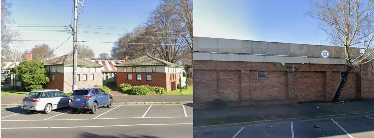
Figure 8: Northern interface (street front)
