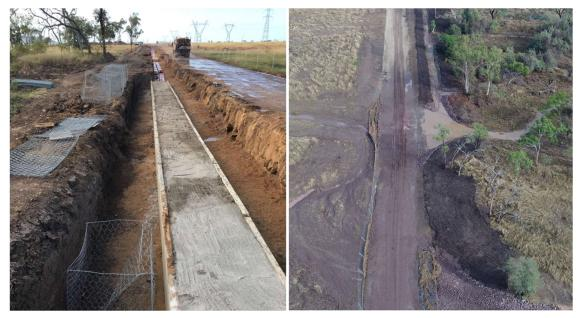
*Figure 13.* Example of a low profile causeway across a watercourse on previous Edify projects (left) under construction and (right) following rainfall.
