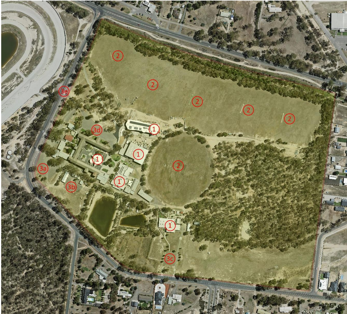
Figure 2-4 Aerial photo of subject site showing location of key assets (photo courtesy of CoGB)
