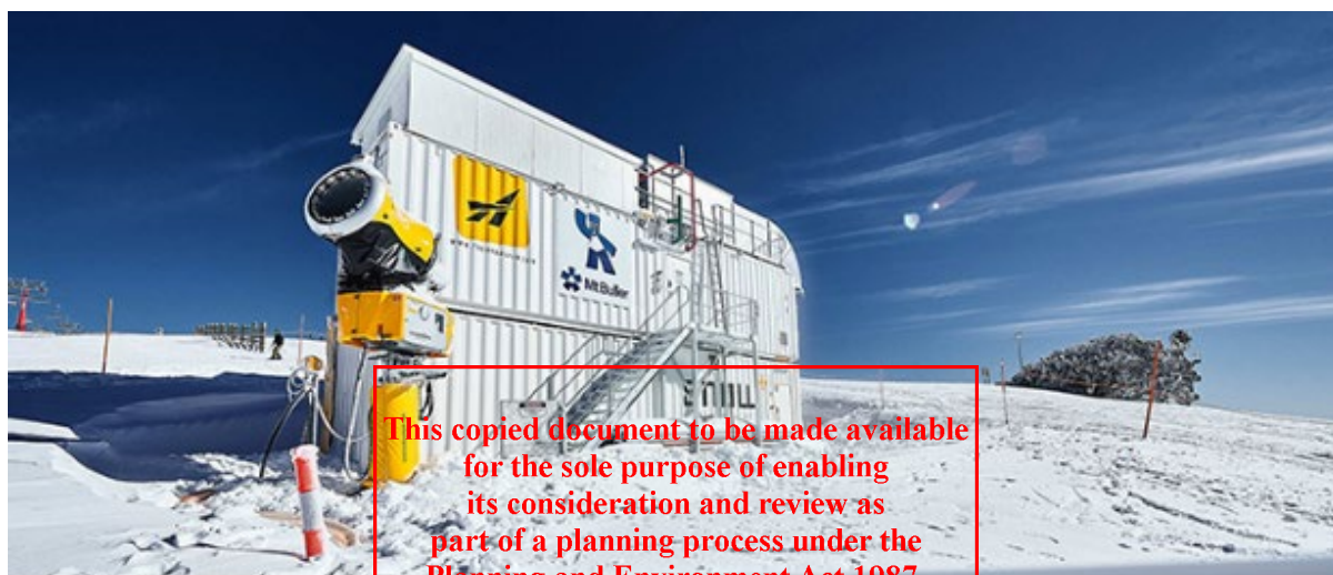
Figure 1: Snow factory, typical installation using 40' modified containers.
