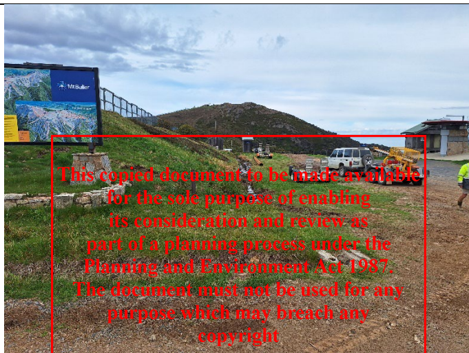
Photo 8: view west along reservoir batter. Note drain along toe
