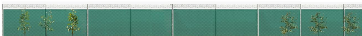
Figure 9 Typical 5m wide screening section – 2 years post installation showing security fence with indicative shade cloth behind
