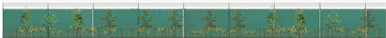
Figure 7 Typical 10m wide screening section - 2 years post installation showing security fence with indicative shade cloth behind
