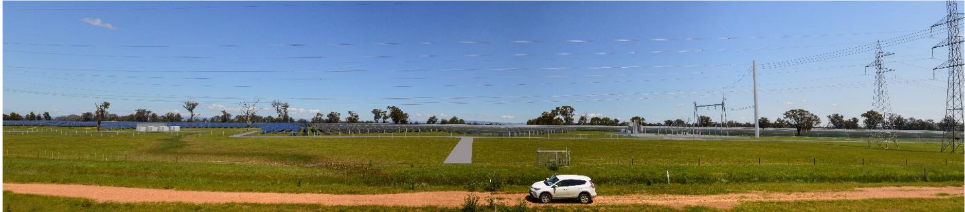
Figure 28 View of Project site along Dam Wall before screening
