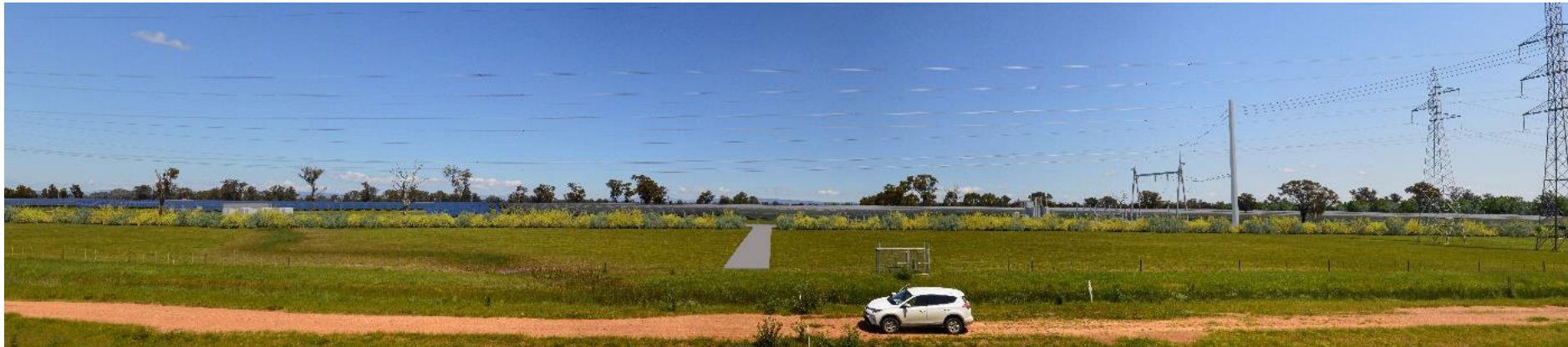
Figure 29 View of Project site along Dam Wall after screening
