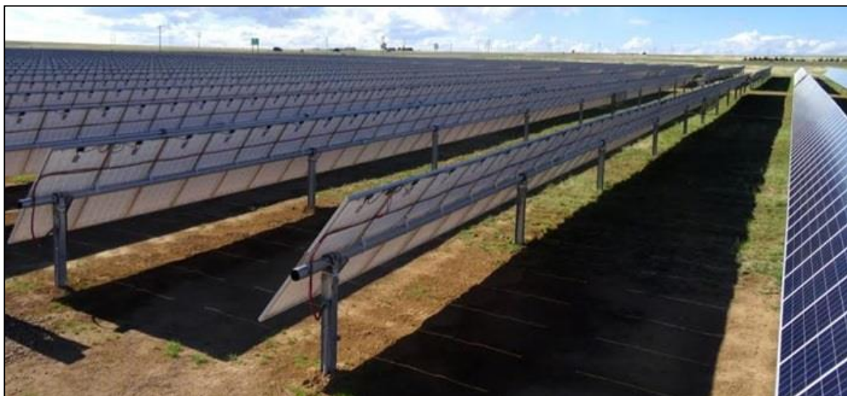
Figure 3-1 Typical Single Axis Tracking System
