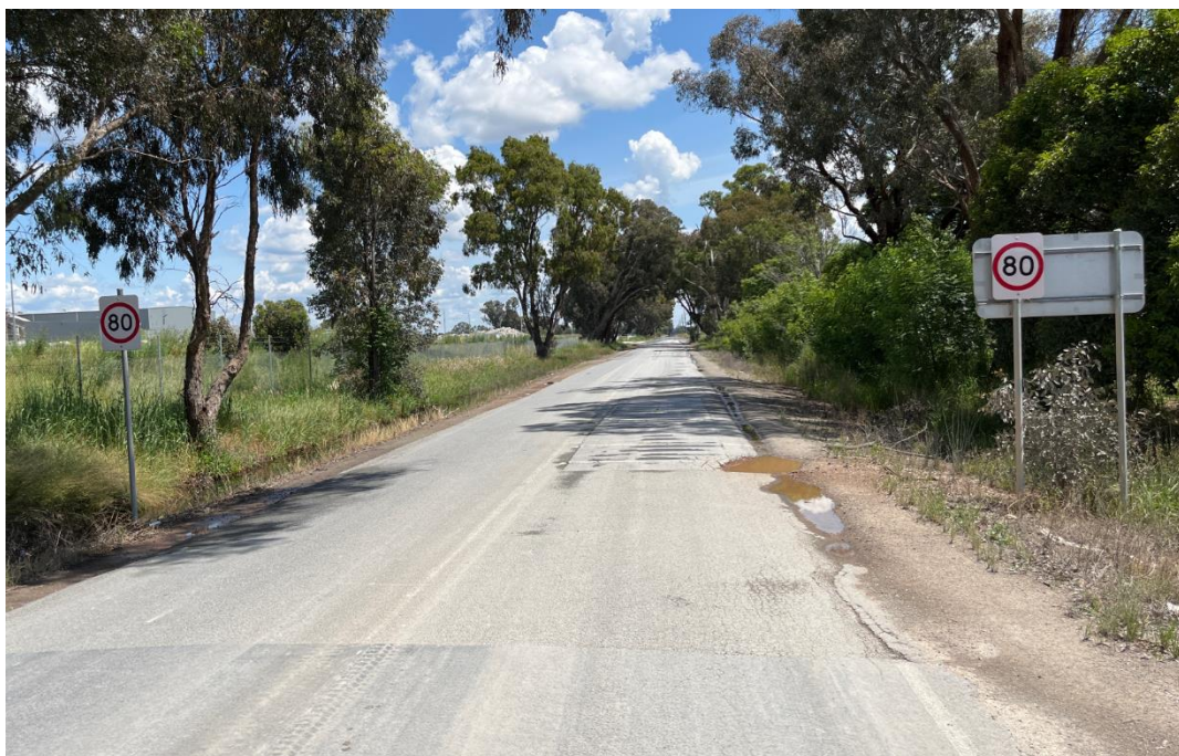
Source: AECOM – photo taken on Wednesday 9 November 2022
