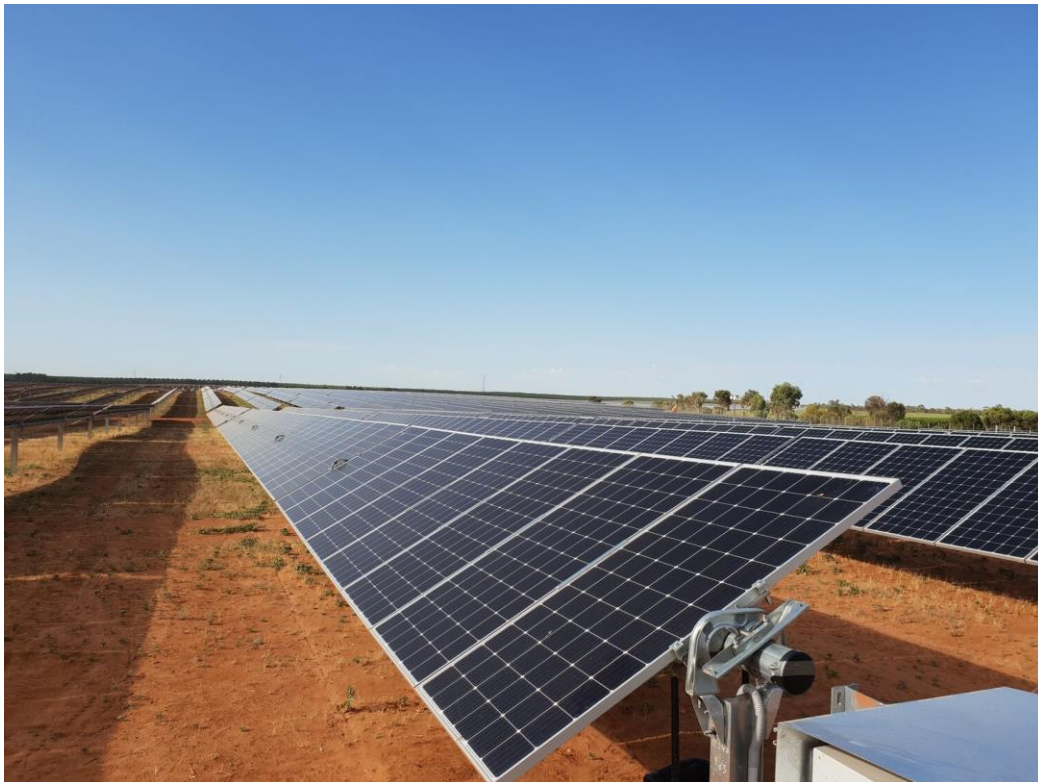
Figure 3-1 Typical Single Axis Tracking System with two modules in portrait orientation
