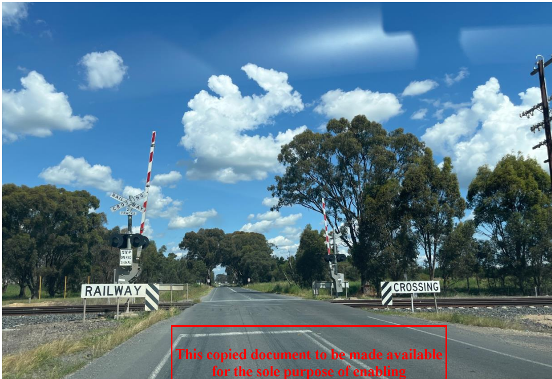
Source: AECOM – photo taken on Wednesday 11 November 2022
