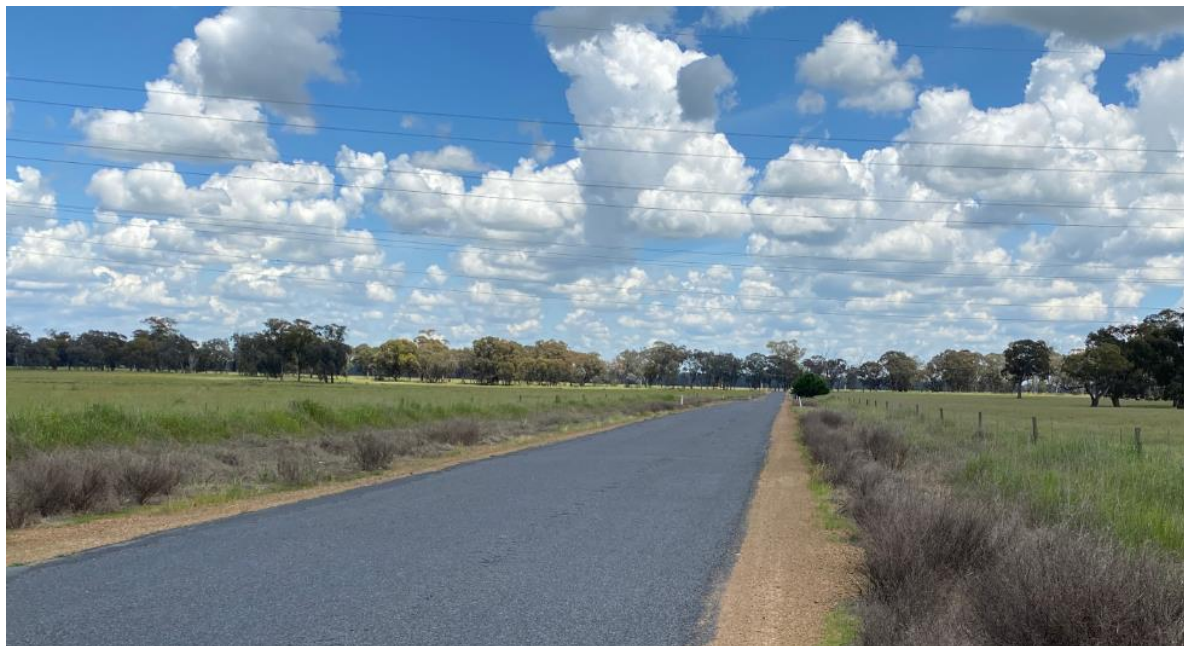
Figure 2-5 Lake Mokoan Road looking westbound
