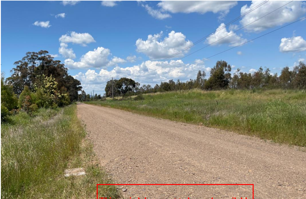
Source: AECOM – photo taken on Wednesday 9 November 2022
