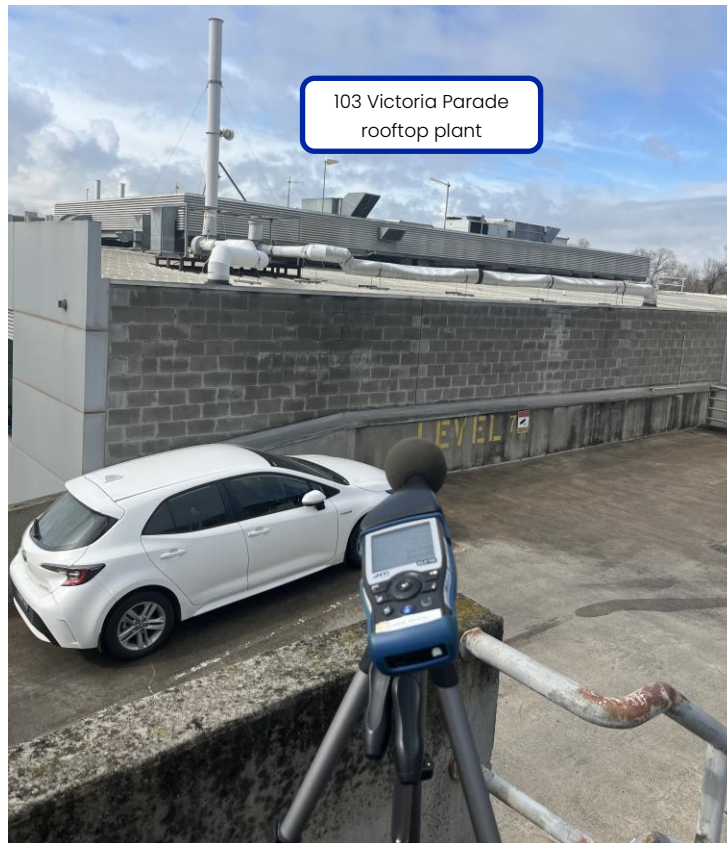
Figure 2 – Attended Measurement Location 1 – 103 Victoria Parade Rooftop Plant
