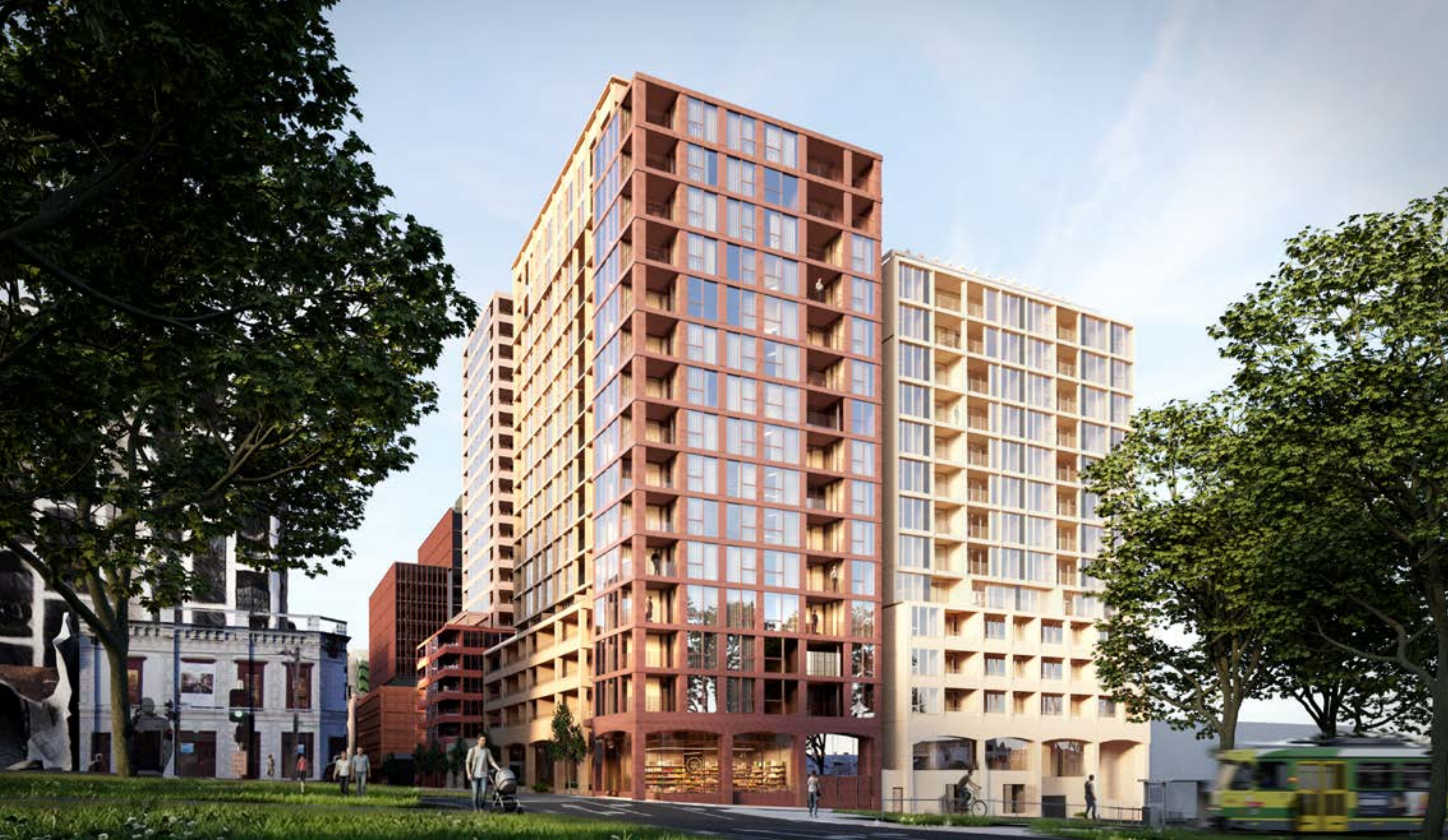
Looking North across Victoria Parade Architectural image, indicative only
