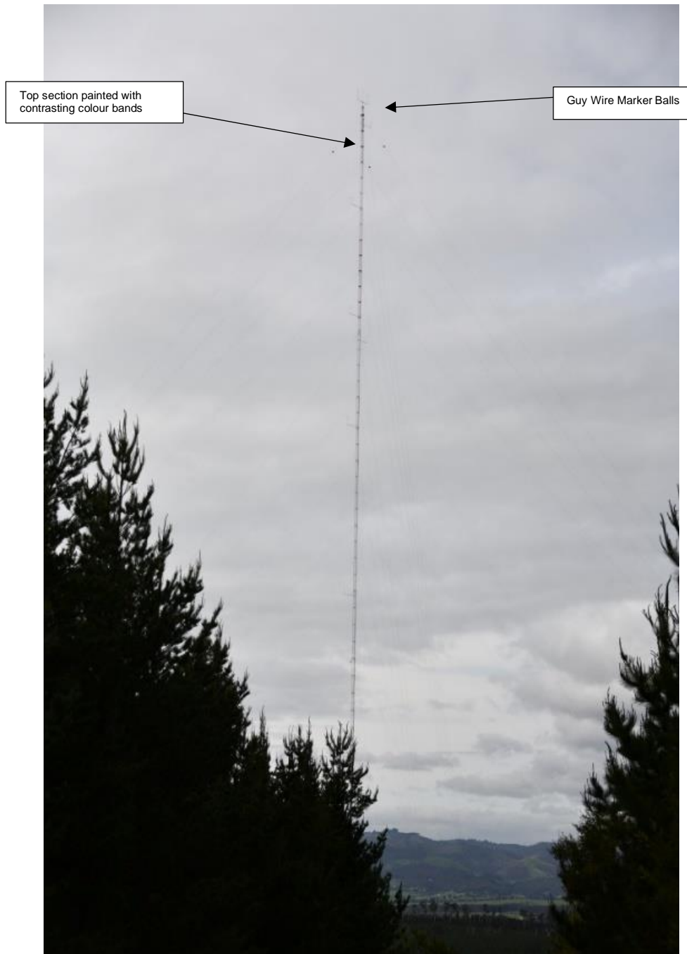
Figure 8 – A Meteorological Monitoring Mast
