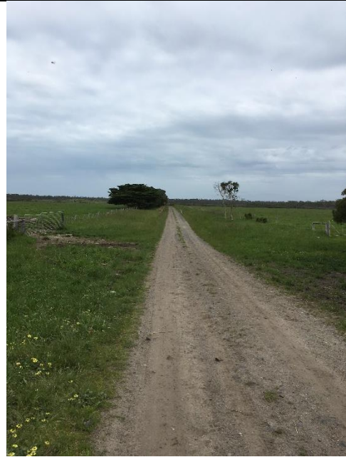
Figure 6 - Typical lower order road located between farms within the Study Area
