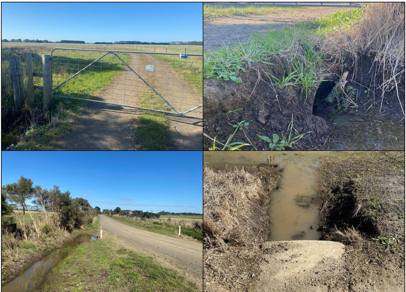
Figure 1-32 Site No. 12 – Inspection Images
