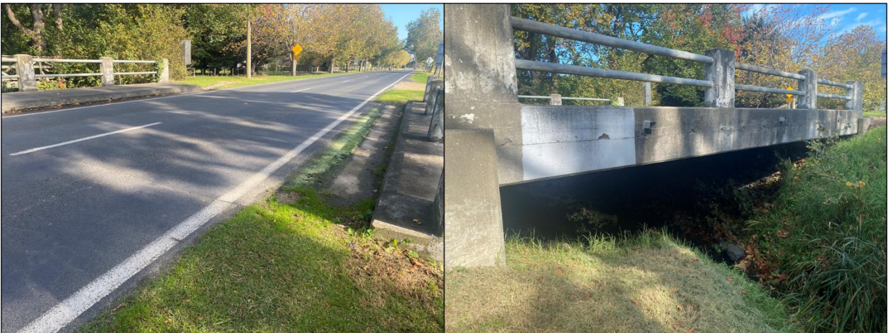
Figure 1-13 Site No. 4 – Inspection Images
