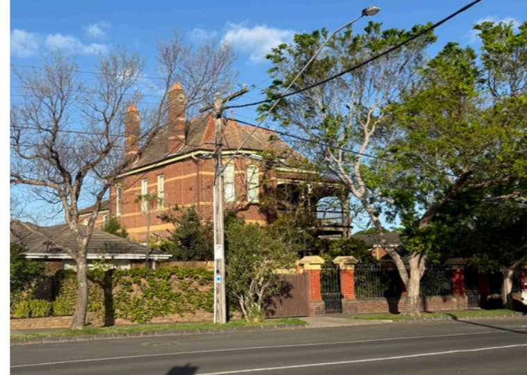
66 Wilson Street 3 Storey brick dwelling
