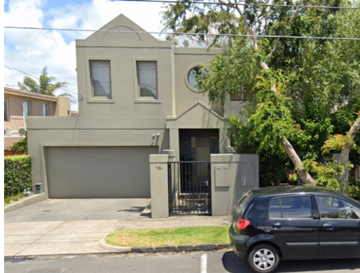
78a Wilson Street 2 storey brick & rendered townhomes
