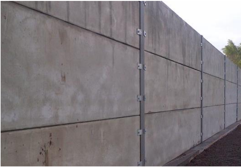
Plate 2.8 Typical acoustic barrier - precast concrete panels (indicative)
