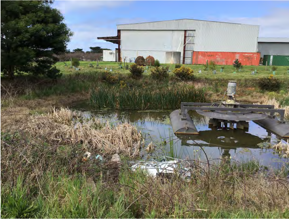
Photograph B.3 View south across Dam 3, adjacent property to the south in the background
