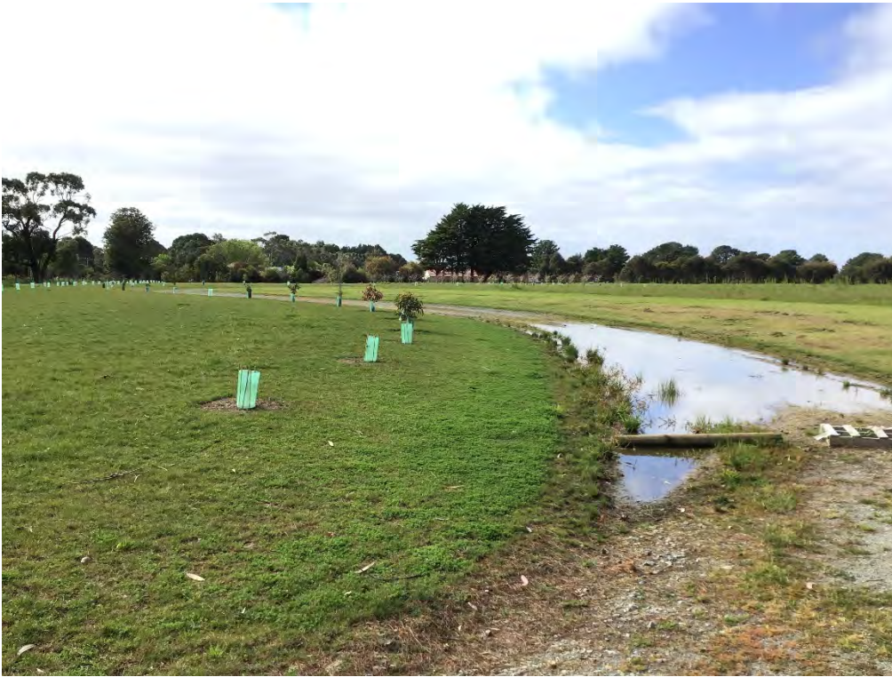
Photograph B.9 Ponding in trapped low point on access track at northern end of site
